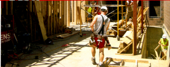
Stevens Construction Corp. crews install a new steel structure inside the façade of an 85-year-old building at 408 W. Gorham St., Madison. The building will soon be home to the Brickhouse BBQ.
